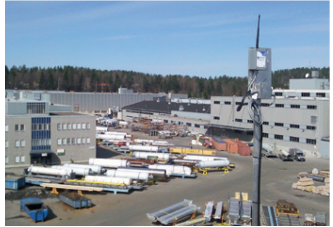
Repeater installation at a paper machine factory
