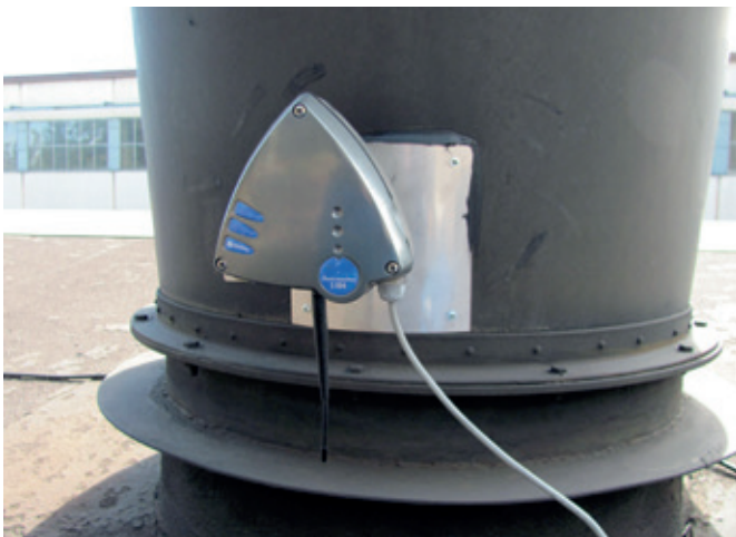
S300 monitor with RF-Link installed at an outlet of a cyclone and at an exhaust stack
